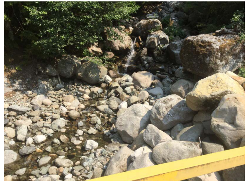
Looking upstream from deck
