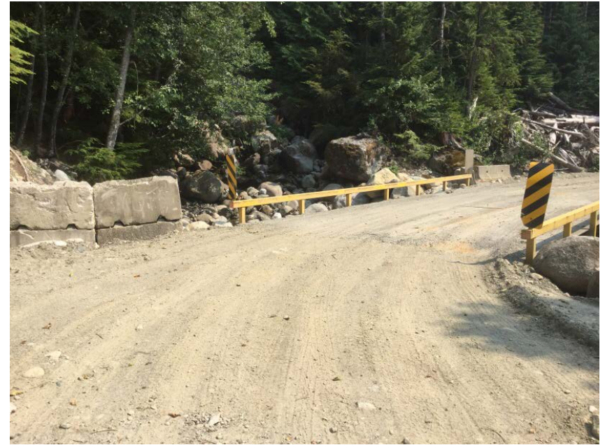
Approach from Right Bank when facing downstream
